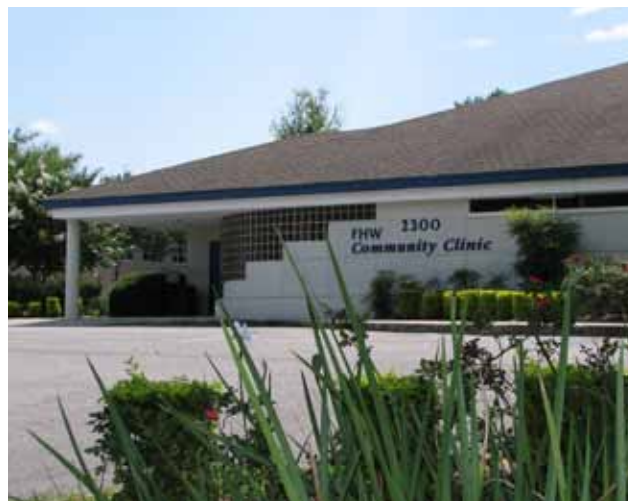
The community clinic building in Eustis provides local residents in need with compassionate care.
