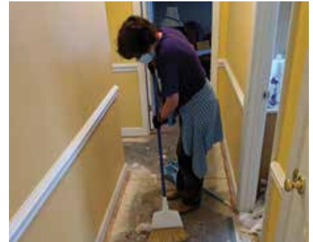
Some flood-damaged houses needed to be gutted, including ripping out carpet and cleaning away debris.
